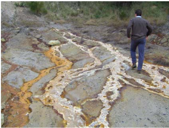
Contaminated Water leaching from side of Adit seal
